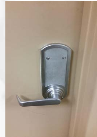
Inside of door
